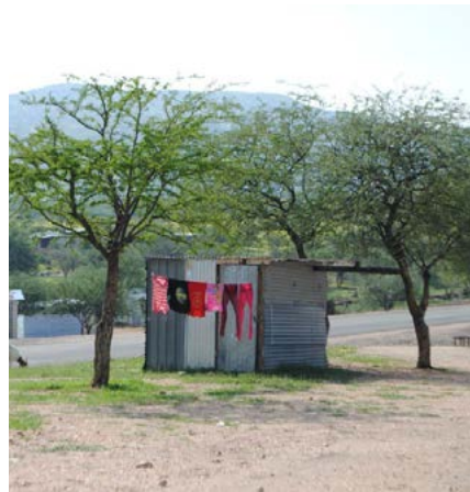
Image 8-9. An 'informal' structure in Namibia.
